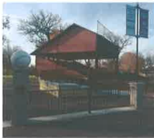
Jones Park Grandstand Renovation & Logo Banners Installed
