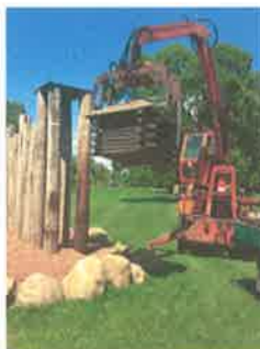
Park Crew/Lions Club constructs 'Welcome' sign in Rock River Park/Hwy 106.
